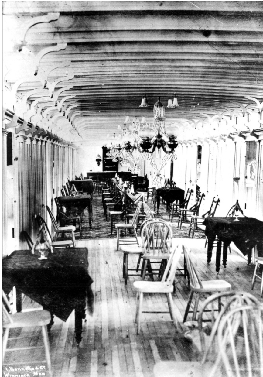
Figure 11 City of Winnipeg, interior. PAM
