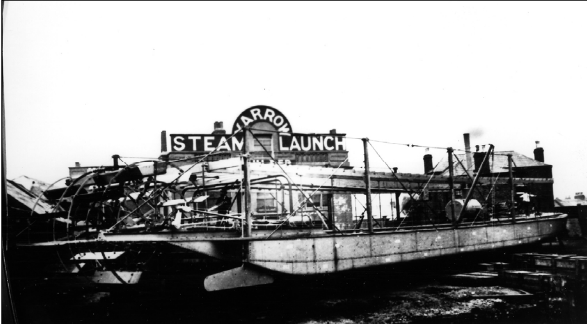
Figure 22 Steel Steamboat under construction Saskatchewan Archives Board Photograph R-B3371
